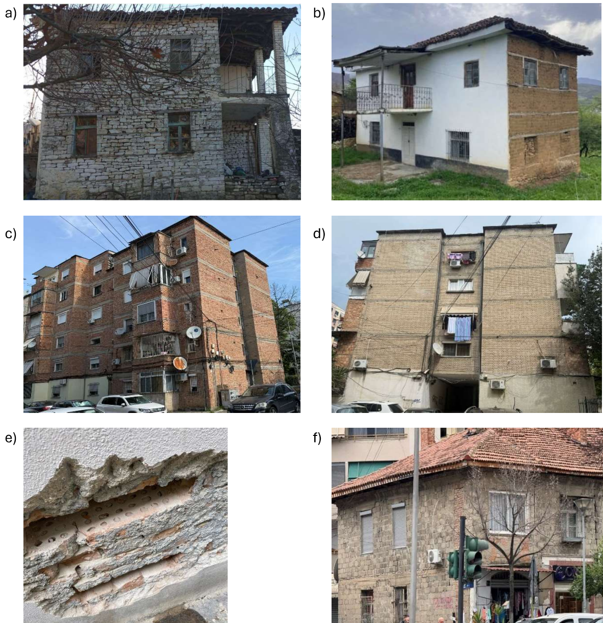
Fig. 44. Masonry buildings with a) stone (regular), b) mud bricks, c) clay bricks, d) silicate bricks, e) hollow bricks, f) concrete blocks
