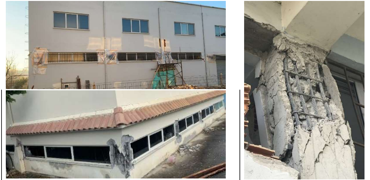
Fig. 28. Captive columns – damaged from Nov. 2019 earthquake
