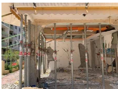
Fig. 65. Example of shoring / propping
