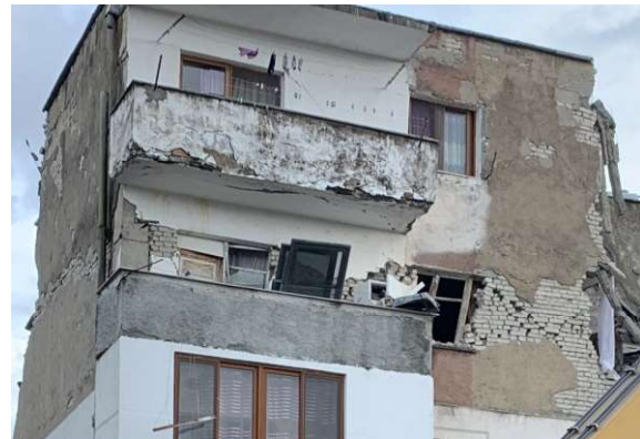
DL extreme: Masonry wall with large displacements
