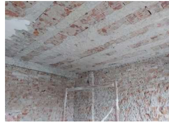
Fig. 15. Floor with prefabricated reinforced hollow clay tile beams with RC ring beams
