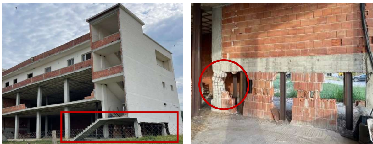
Fig. 27. Short column due to beam of stair landing
