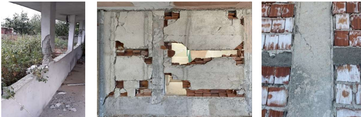
Fig. 29. Left: short column effect. Middle and right: Inappropriate connection RC frame - Tie beam
