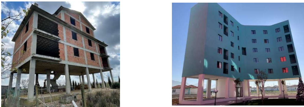
Fig. 22. Existing buildings with irregularities in elevation – soft storey
