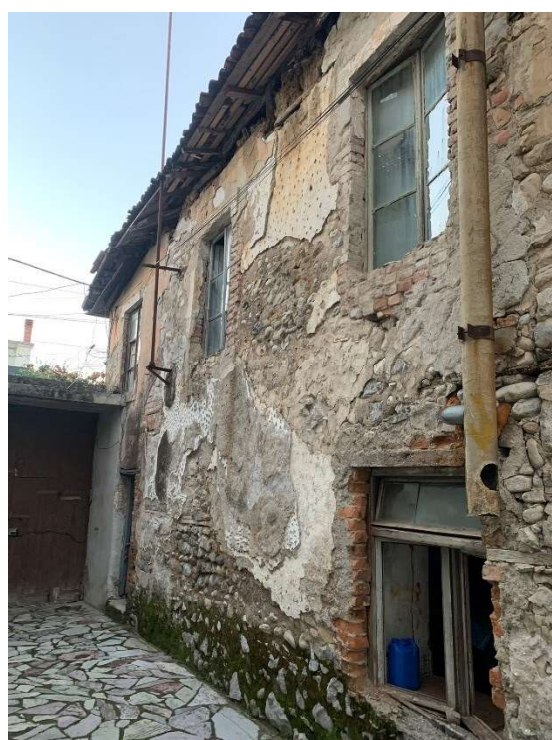
Fig. 37. Example of building with damage due to lack of maintenance
