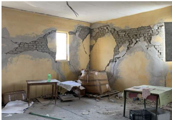
DL Severe: Large cracks at masonry wall
