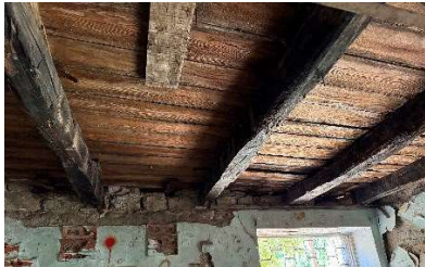
Fig. 14. Wooden flexible floor
