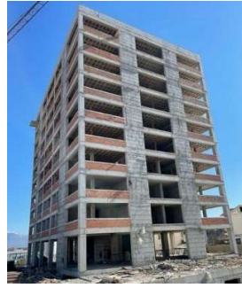
Fig. 49. RC shear wall system
