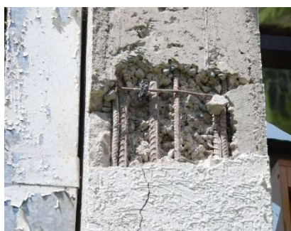
Fig. 31. Low quality of concrete in RC structures
