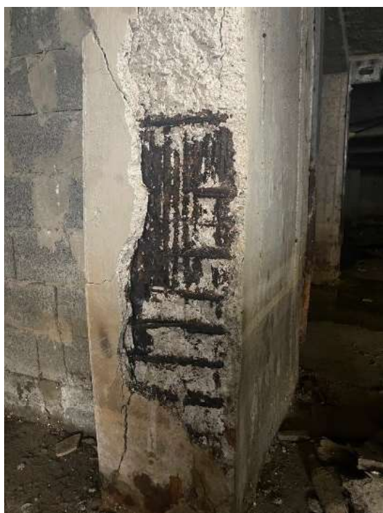
Fig. 36. Example of RC element with rusted and corroded rebars
