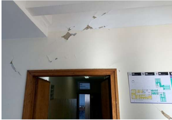
DL light: Shear cracks at the masonry spandrel
