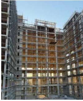
Fig. 48. RC frame system
