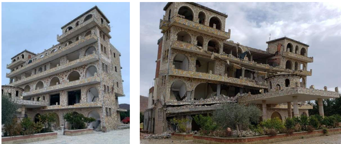
Fig. 6. Left: Damaged building after the Nov. 26, 2019, earthquake in Durrës. Right: same building, with increased damages due aftershock of Jan. 01, 2020 (photo F. Guni)
