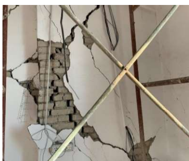
Fig. 30. Cracks in silicate brick masonry showing weak brick-mortar bond
