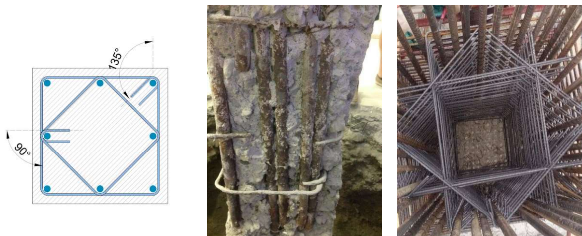
Fig. 34. Left: Closed hoop stirrups as required by KTZ 10/1-1978. Middle: Poor detailing of stirrups. Right: Properly closed hoop stirrups.
