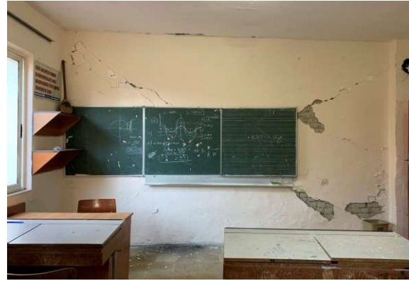
DL Moderate: Shear cracks at masonry wall
