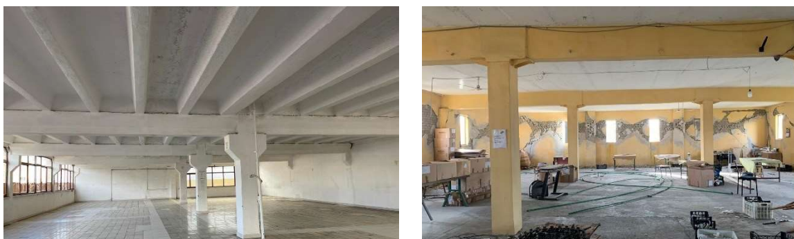
Fig. 19. RC frames in one direction. Left: with prefabricated element. Right: cast in place
