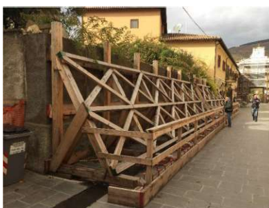
Fig. 65. Example of shoring / propping
