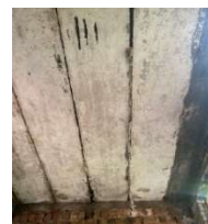
Fig. 17. Prefabricated pretensioned panel
